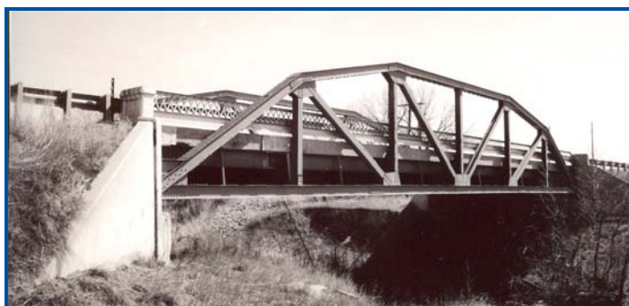
Little Thompson River Bridge
